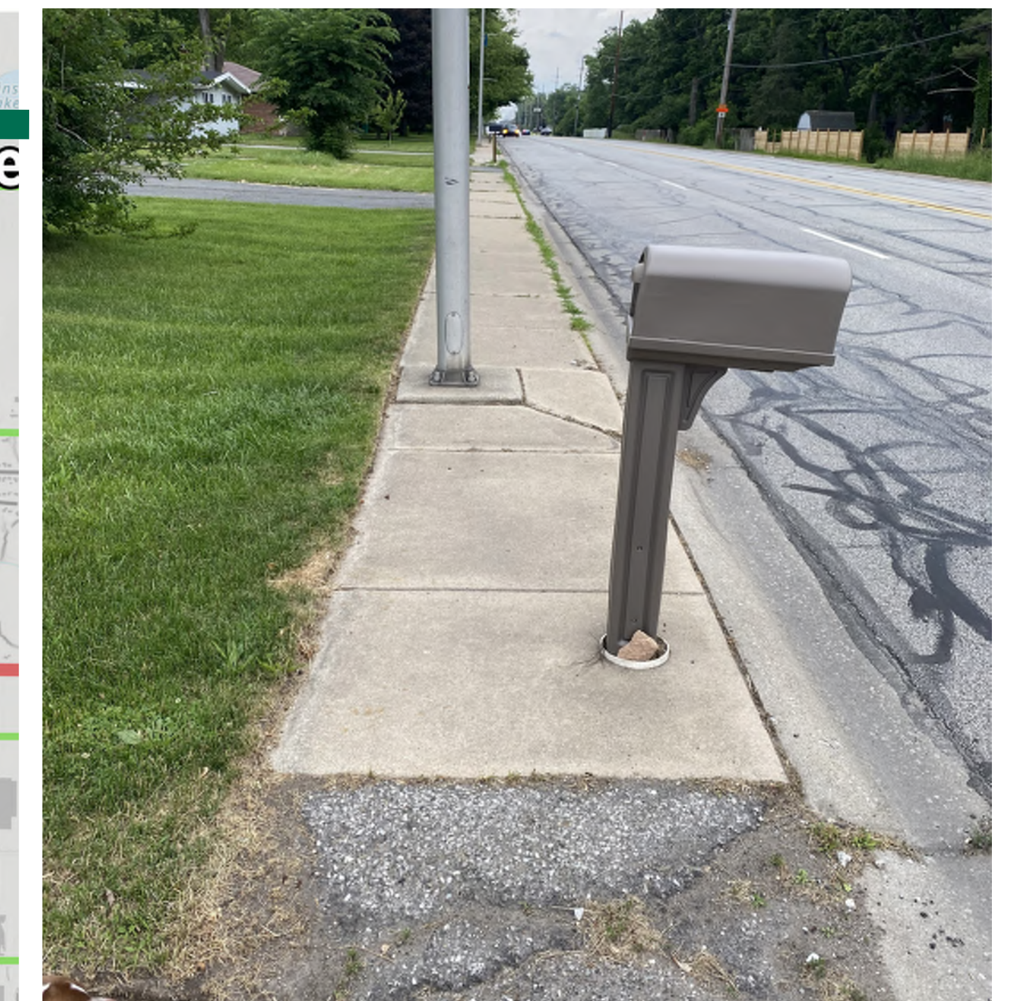
Obstacles on Madison Street. Back of curb sidewalks unbuffered from moving traffic and obstructed by mailboxes and light poles make life difficult for pedestrians.
