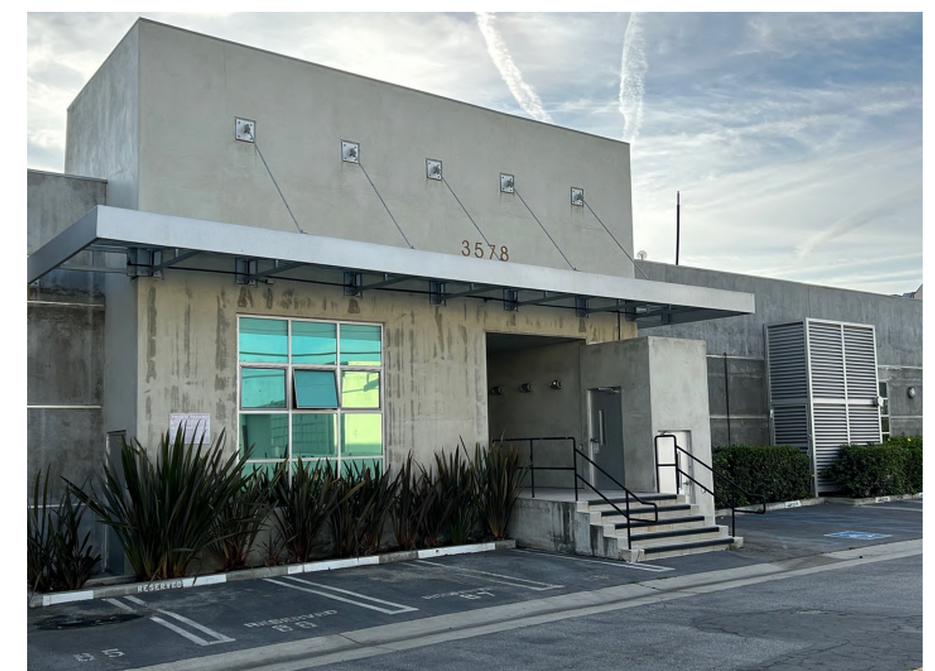
Buildings for innovative start-ups. Hayden Tract in Culver City, CA
