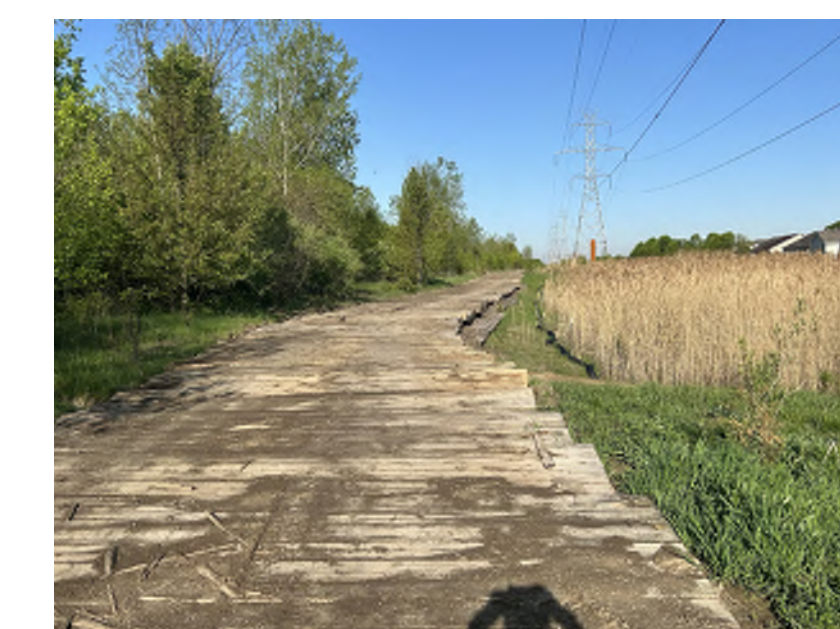
Merrillville Utility Corridor. This corridor presents a major opportunity for connecting neighborhoods and establishing an iconic greenway through the Town's south side.
